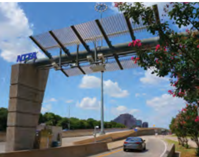
North Texas Tollway Authority Gantry | Dallas, TX
