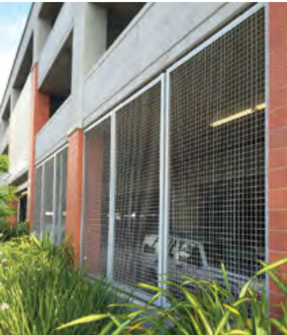
Miramar College Parking Structure | San Diego, CA
