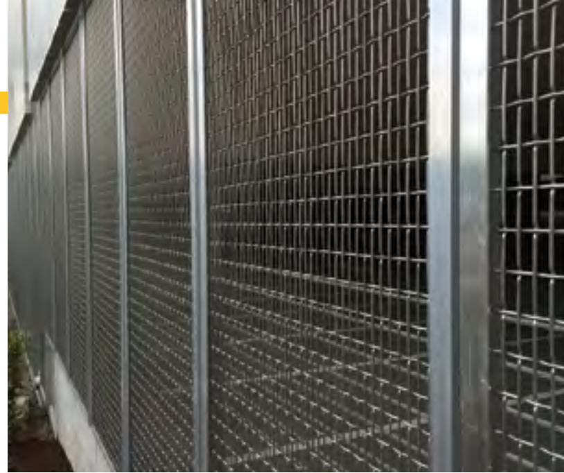
Daimler Trucks North American Parking Structure | Portland, OR
