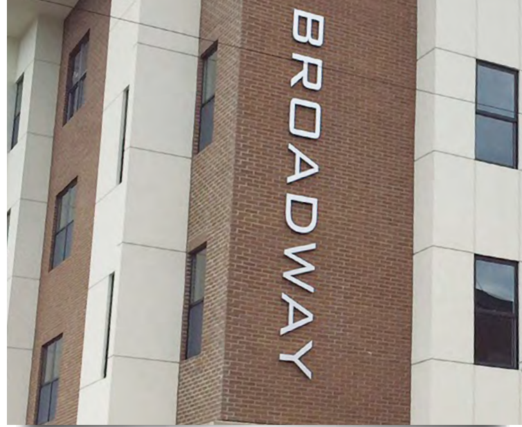
Office Building Schenectady, NY
